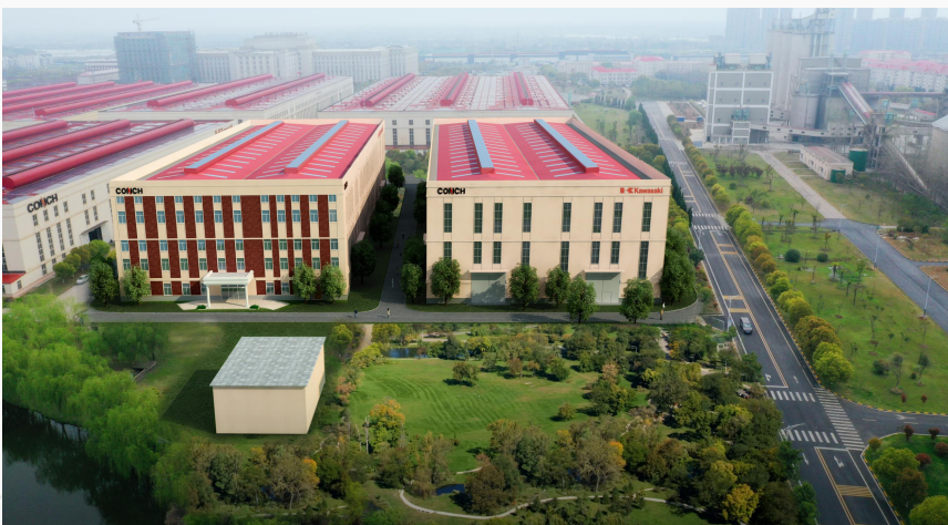
Aerial view of China's first set of cement kilns to treat waste lithium batteries
