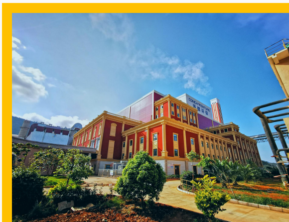
Project in Baoshan-Yunnan
